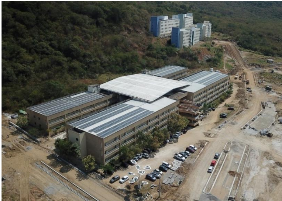
Figure 3.3 Rooftop solar plant at the Auroras Campus (UNILAB).
